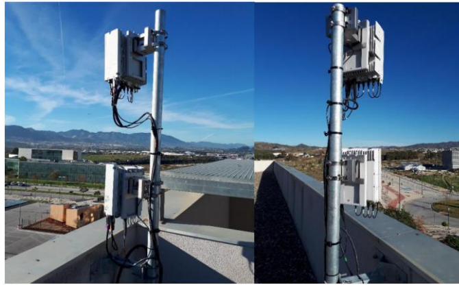
Figure 56: Nokia 5G and 4G micro RRH in Ada Byron building rooftop
