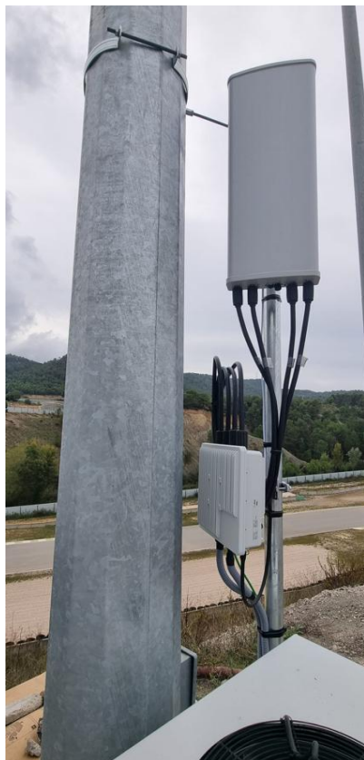
Figure 57: Node #9 RAN installation
